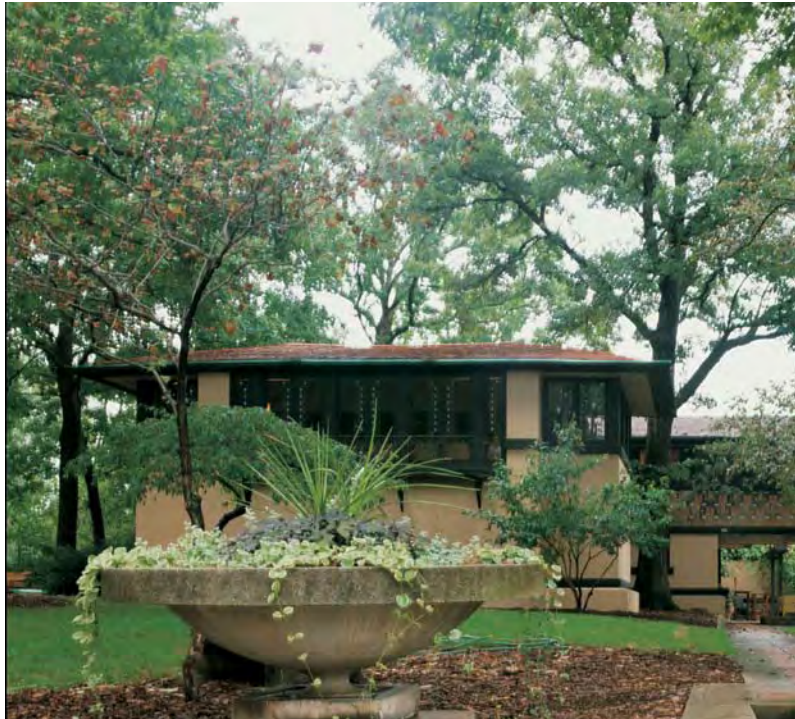
The Avery and Queene Coonley House - Riverside, Illinois - 1907. Situated along the Des Plaines River, the Coonley House is the largest and most expensive of all Wright's Prairie Houses. Both clients were business fortune heirs. Wright designed all the features and furnishings within the home, including rugs and textiles. The plan is unique in Wright's Prairie style houses; the various components of the plan are zoned. One second-floor zone includes the living room and dining room, another, the bedrooms. A third zone containing the kitchen and service areas connects to the dining room. The living room, playroom, and entrance hall are on the ground floor.
