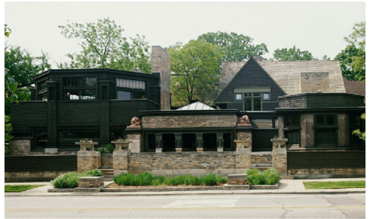
Studio Addition to the Oak Park Home-1897
